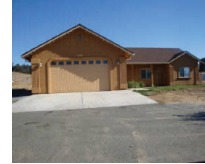
Valley Springs 3671 Highway 26 $169,900 #102336
